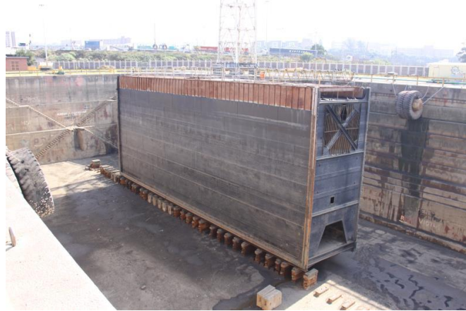
FIGURE 3 CAISSON IN GRAVING DOCK [2]
