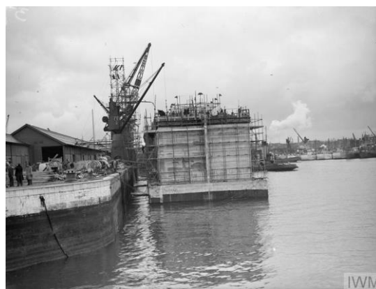
FIGURE 4 CONSTRUCTION AT QUAY SIDE [3]
