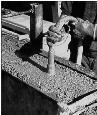
FIGURE 63 COMPACTION OF CONCRETE [12]
